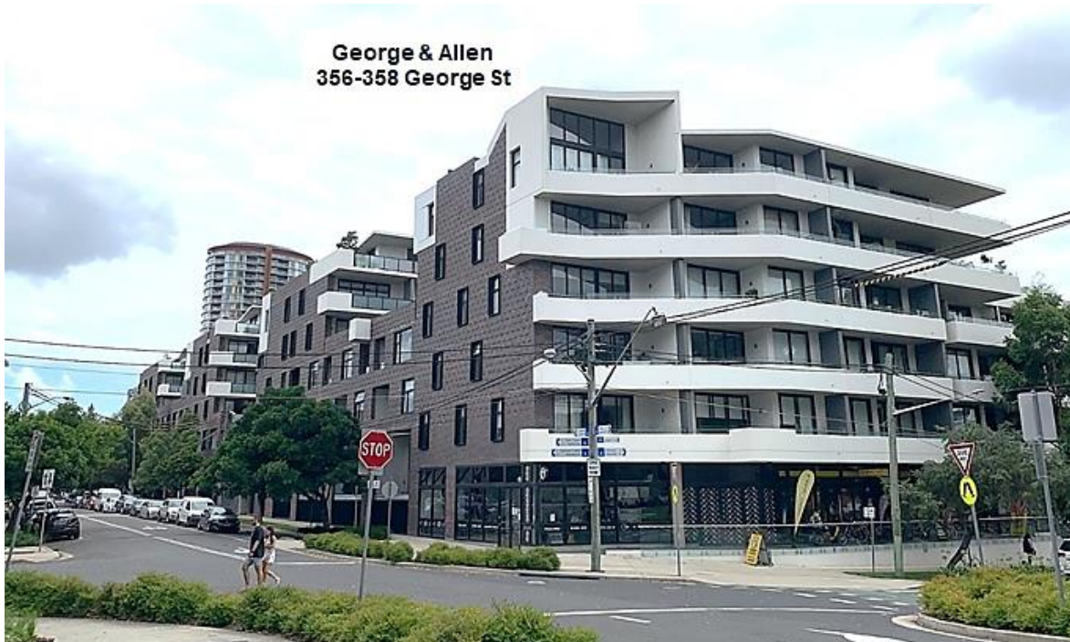
Figure 7: 'George and Allen' buildings at 356-358 George Street Waterloo, north-east of the subject site
