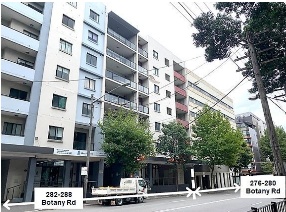
Figure 13: Mixed-use building at 282-288 Botany Road Waterloo on the opposite / western side of Botany Road
