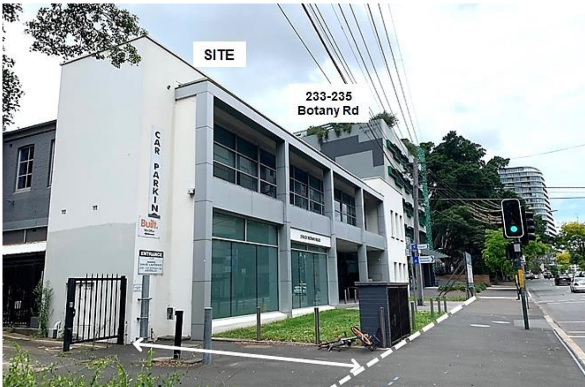
Figure 3: Subject site looking south with arrow indicating strip of land to be dedicated in accordance with VPA
