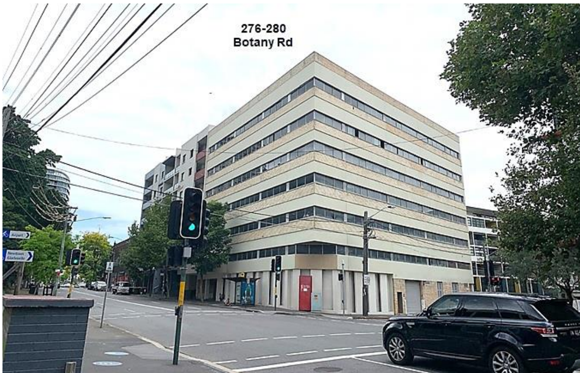
Figure 11: Commercial building at 276-280 Botany Road Waterloo on the opposite south-western corner of Botany Road and Mandible Street
