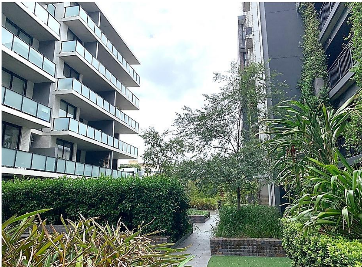
Figure 8: View from one of the podium-level courtyards of the 'George and Allen' building towards the subject site to the west
